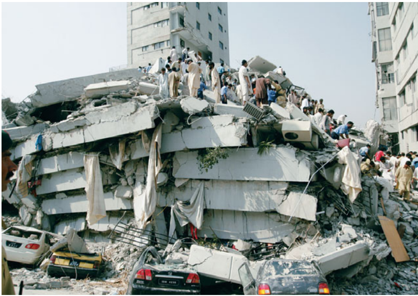
◀ FIGURE 1.3 DEVASTATING EARTHQUAKE People search for victims in the rubble of a 10-storey building in Islamabad, Pakistan, that collapsed during a large earthquake in 2005. About 86 000 people died and 3 million more were left homeless. (Warrick Page/Getty Images)
