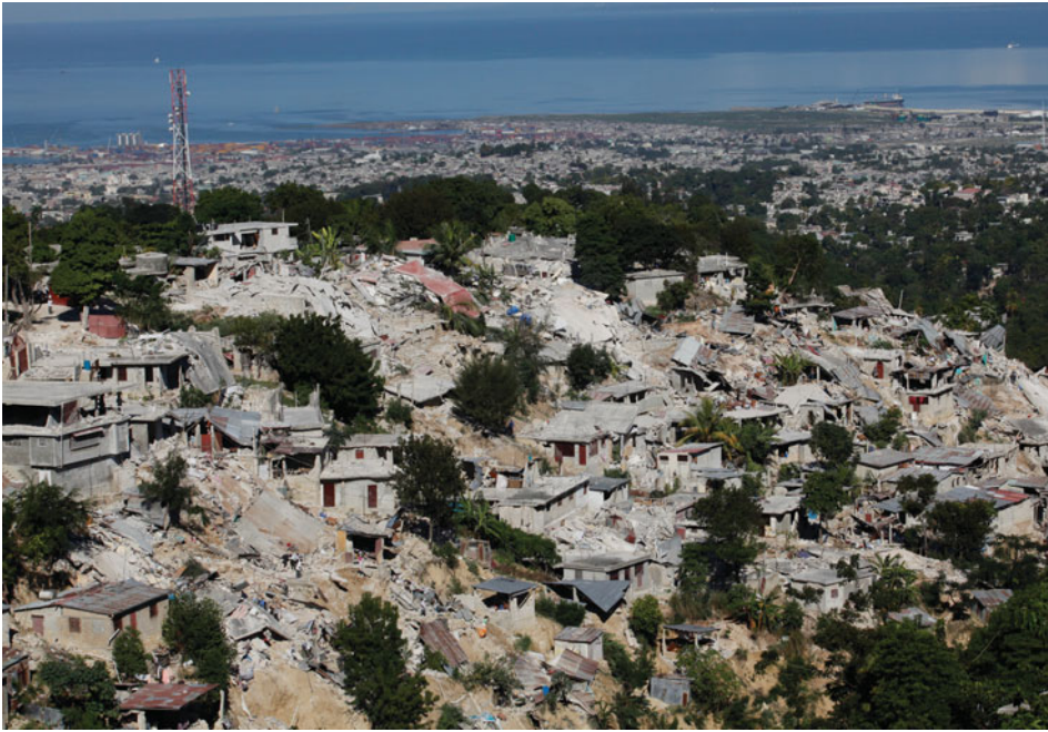
◀ FIGURE 1.1 EARTHQUAKE DEVASTATION IN HAITI Unreinforced and poorly reinforced masonry and concrete slab buildings in Canapé Vert, a shantytown in the hills around Port-au-Prince, collapsed during the January 12, 2010, earthquake ( Eduardo Munoz/Landov )
